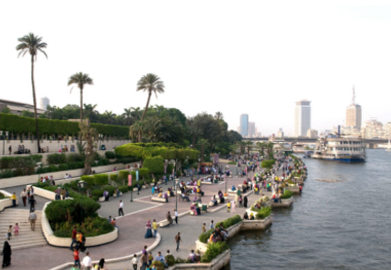
Fig. 2.10: Ahl Misr walkway after construction.
