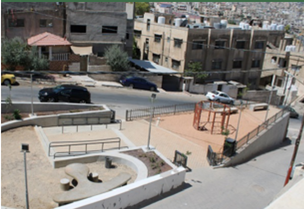
Fig. 3.1: The Seventh Stair on Al-Quds Street after rehabilitation works.
