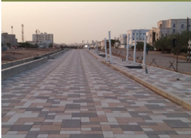
Fig. 3.71: The project under implementation phases.
