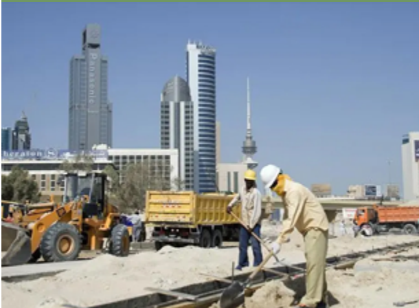
Fig. 3.32: Construction workers on site.
