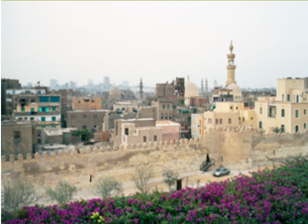
Fig. 3.92: Houses in Darb al-Ahmar after the intervention.
