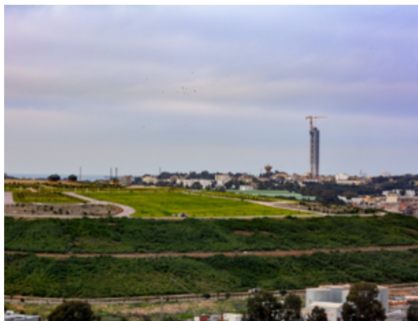
Fig. 3.91: Aerial view showing the Oued Smar Urban Park after implementation.
