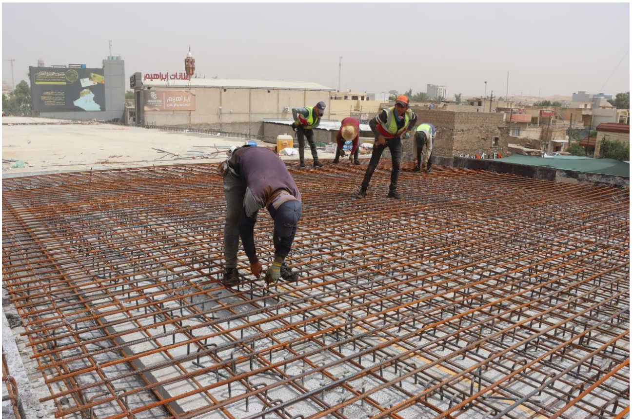
Construction of the second lane of the Sennacherib flyover intersection ©2025 Municipality of Mosul
