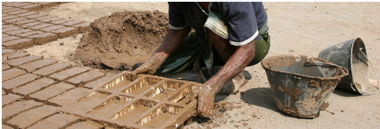
Reconstruction work for the Project for the Development of Historic Cities in Yemen ©2004-2007 NNDDesign Studio | GIZ Yemen
