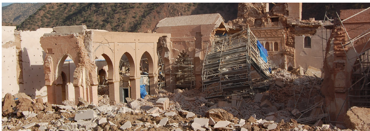
Damages on Tinmel Mosque after the 2023 earthquake in Morocco ©2023 Lucyin | Wikimedia Commons
