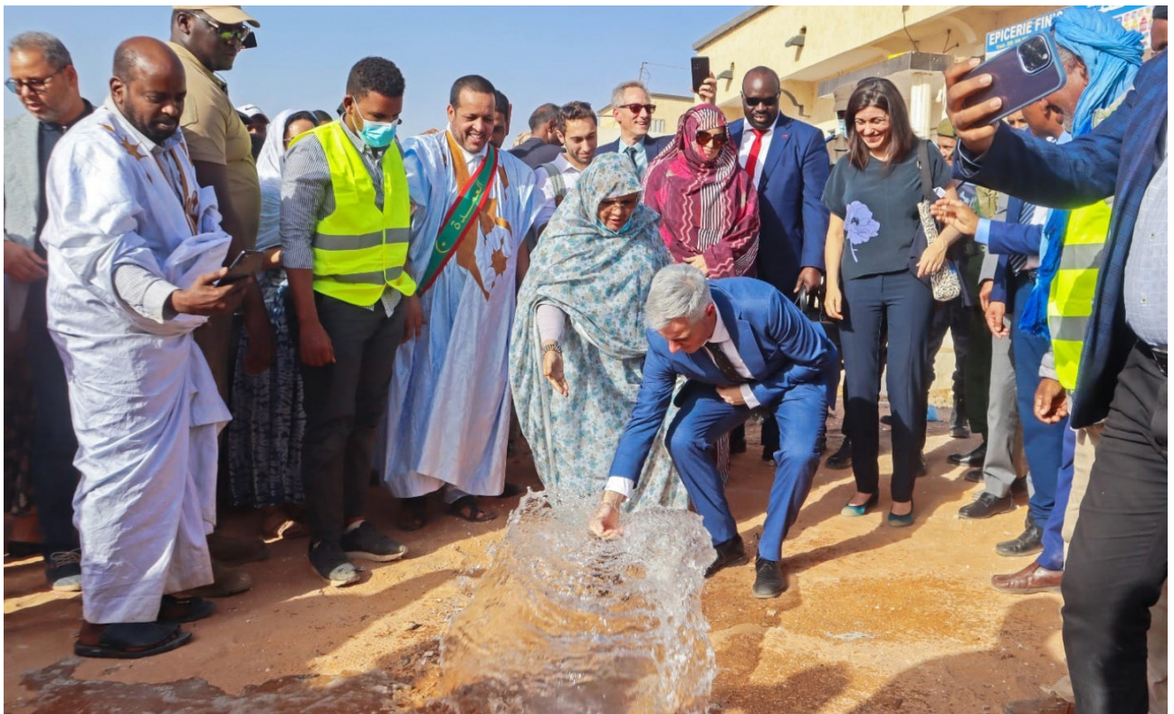
Inauguration of a new 21km pipeline in Nouakchott during the visit of a Swiss delegation ©2024 Ville de Lausanne
