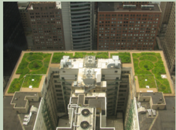
Figure 12.1: The green roof at the city hall of Chicago
