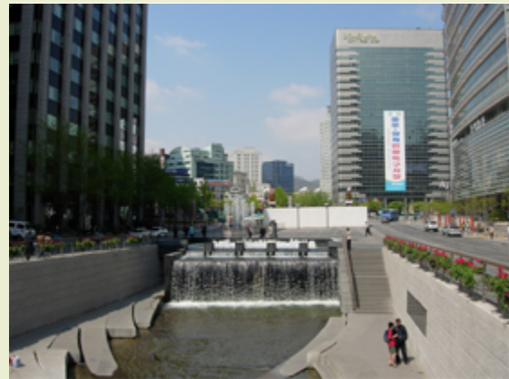
Figure 7.4: The Cheonggyecheon Stream Restoration Project © W00kie, 2006
