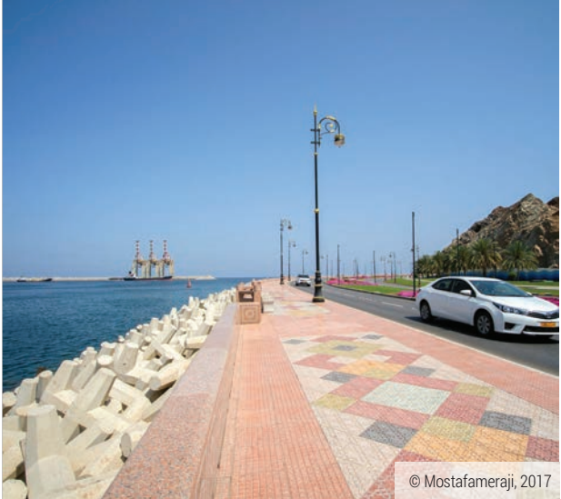
Figure 4.7: A newly constructed walkway, part of Oman Vision 2040's Infrastructure Enhancement and Development Projects
