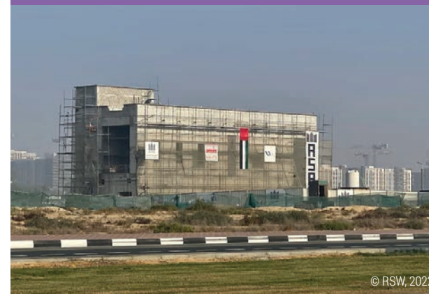
Figure 4.95: Construction of the container depot is completed in 2022.
