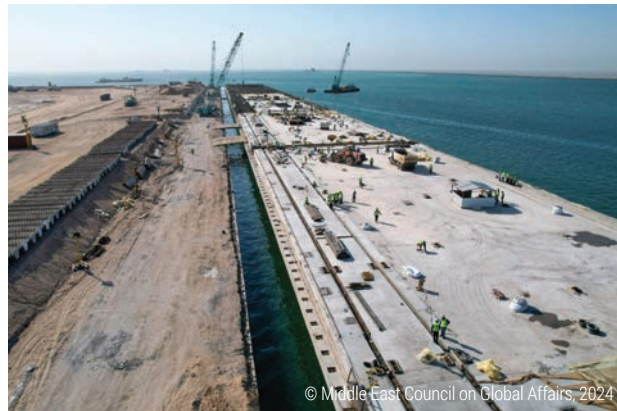
Figure 4.38: Construction of Iraq's Development Road Project.
