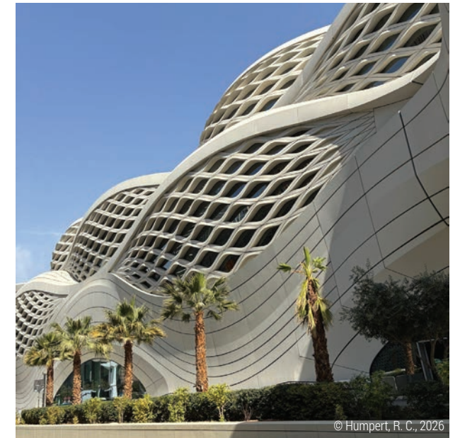
Figure 4.72: King Abdullah Financial District (KAFD) metro station.
